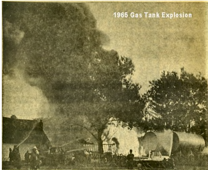
Figure 5.4.5-4. 1965 Gas Tank Explosion
